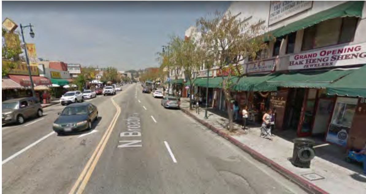
Lack of visual cue for the lane shift on Northbound N. Broadway. The closest vehicle on the left side of the street is parked in the red zone (Source: Google Streetview)
