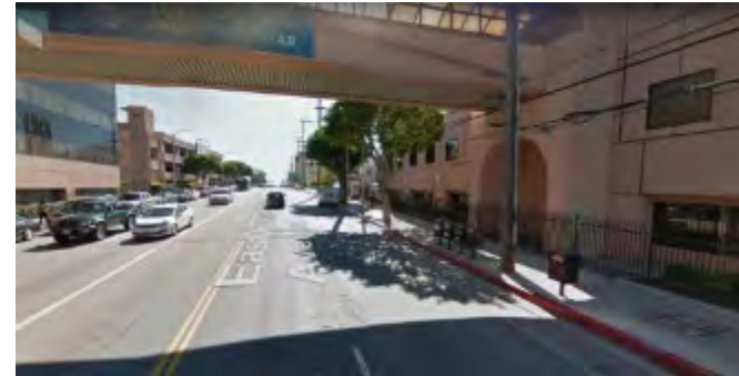
Westbound approach to the White Memorial Medical Plaza with no directional signage to the parking area, and with a vestigial
