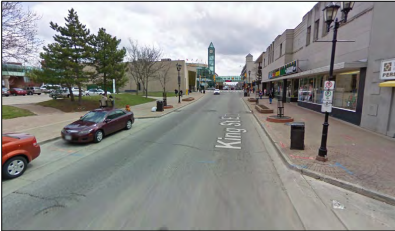
Before construction (above) with inflexible curb space and after construction (below) with removable bollards
