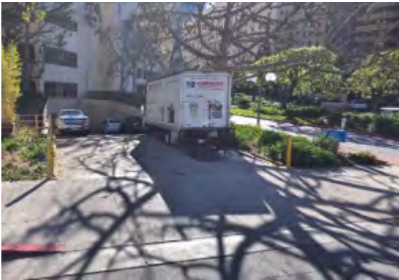
Good Samaritan Hospital loading dock filled with personal vehicles and a delivery vehicle in February 2018. Source: Google Streetview
