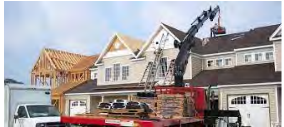
Exhibit 2-20: Roofing Delivery Truck
