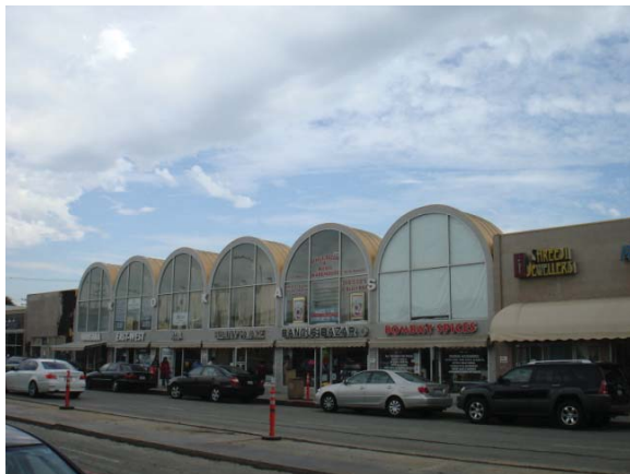
A mix of commercial retail along Pioneer Avenue contributes to the visual character of Little India.
