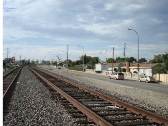
Several single family homes adjacent to the tracks through South Gate, Cudahy, and Bell.
