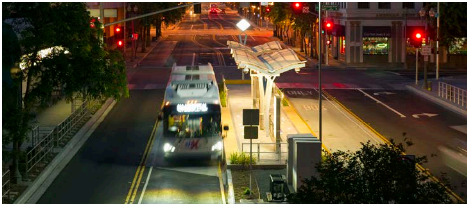
SbX with its bus-only lanes in downtown San Bernardino, CA
