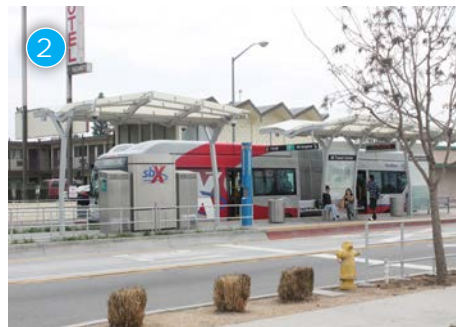
View of the sbX stop at the E/Rialto intersection
