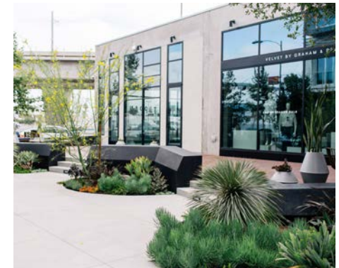
Platform, Culver City, CA
