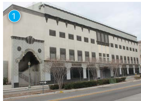
View of the historic Harris Building on E Street
