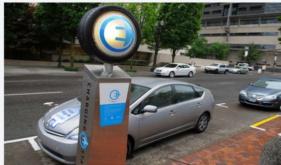
Curbside electric Vehicle charging station, Portland, OR
