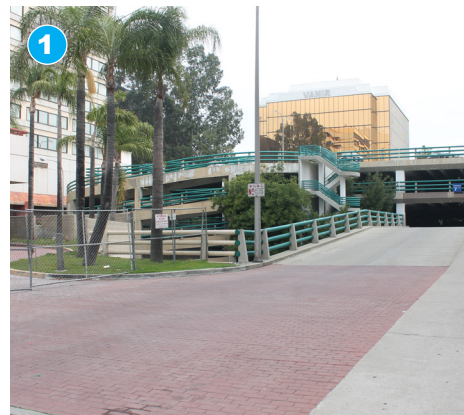
View of the Civic Center parking structure
