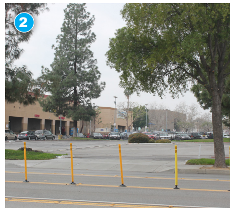
View of the existing retail along E Street
