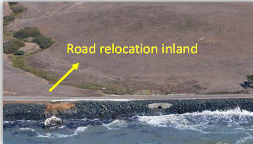
Figure 22. Photo depicting planned retreat for major public infrastructure. The Piedras Blancas Highway 1 Realignment will move nearly 3 miles (5km) of Highway 1 500 ft (152 m) inland. (Source: California Coastal Records Project )
