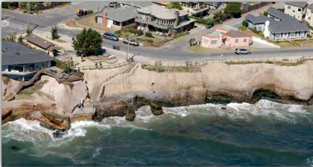
Figure 25. Photo depicting protection of visual resources and public access. A seawall visually blends in with the natural bluff while surfing access is also provided at Pleasure Point, Santa Cruz (2013). (Source: California Coastal Records Project )
