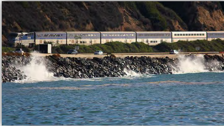
Figure 7. Photo of infrastructure at risk near Rincon Beach, Ventura, CA, during the King Tide in December 2012. (Photo courtesy of David Powdrell, California King Tides Initiative)
