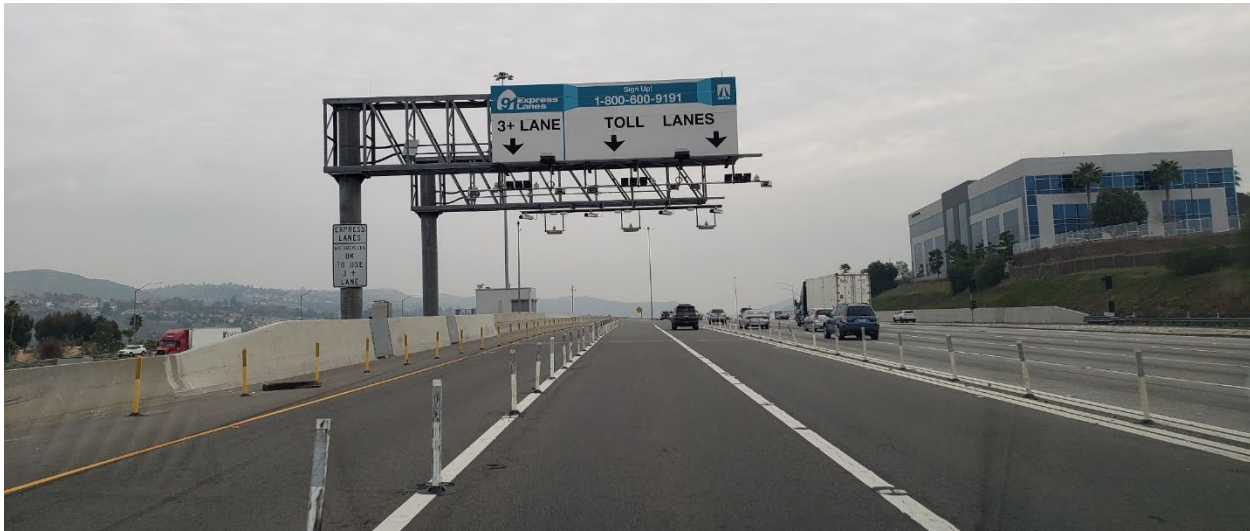
Figure 6-1. Declaration Lanes on 91 Express Lanes in Orange County
