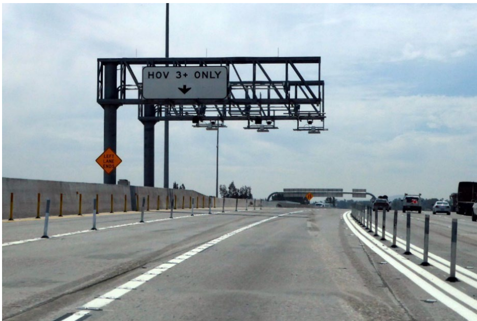
Figure 5-4. SR-91 Express Lanes in Orange County with Channelizer Separation
