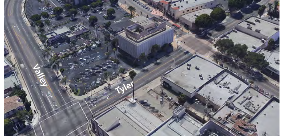
E Tyler Ave / Valley Mall - Valley Blvd
