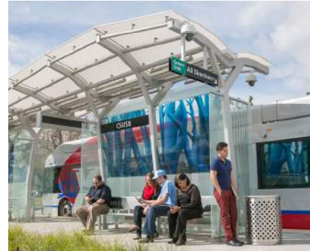
sbX Transit Shelter, San Bernardino, CA
