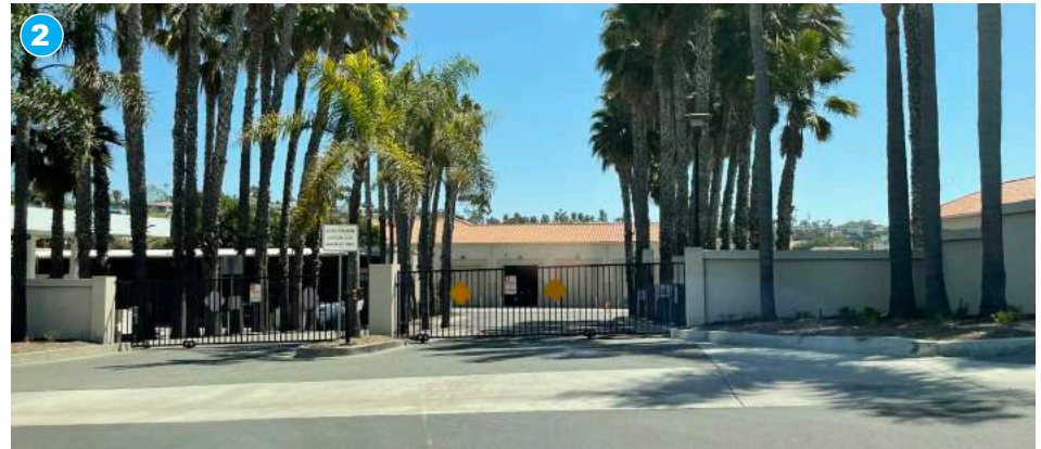
Water reclamation plant
