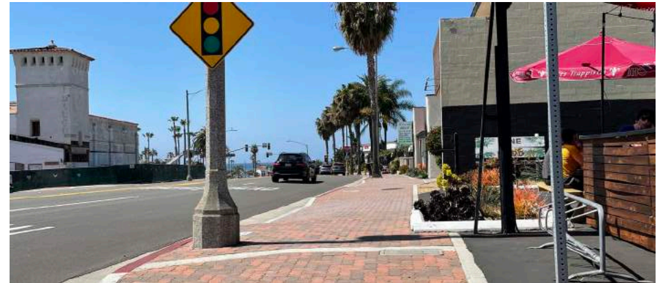
Existing Condition: Decorated/brick sidewalk paving
