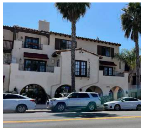
Architectural character of area
