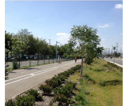
Orange Line Busway, Chatsworth, CA
