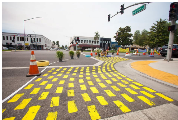
Temporary Yellow Brick Road Curb Extension
