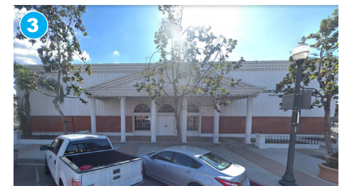
Historic/unique facade in Downtown
