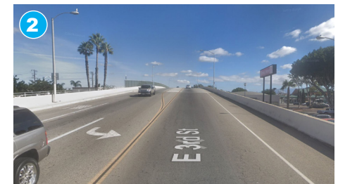
3rd Street Bridge
