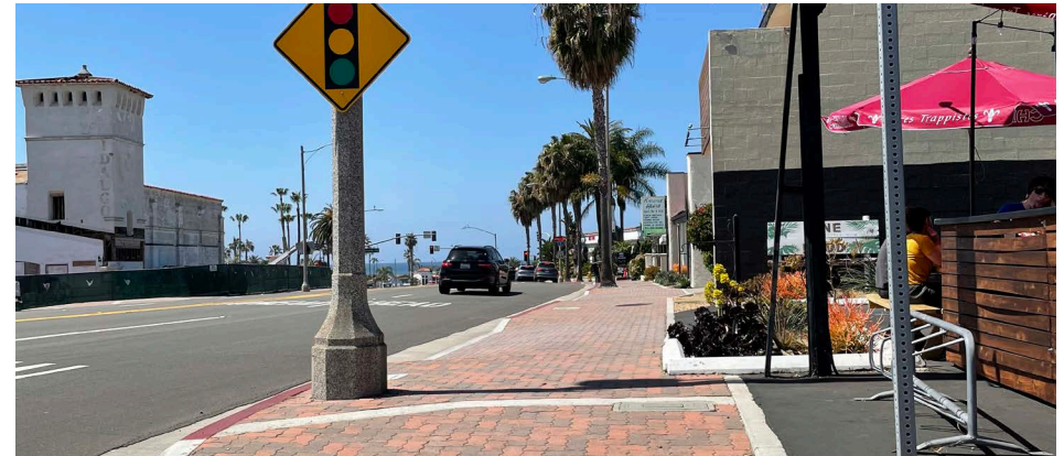
Existing Condition: Decorated/brick sidewalk paving
