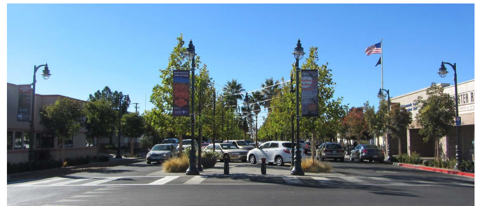
Example roadway with a single lane of traffic in each direction, on-street parking, and a flexible center median
