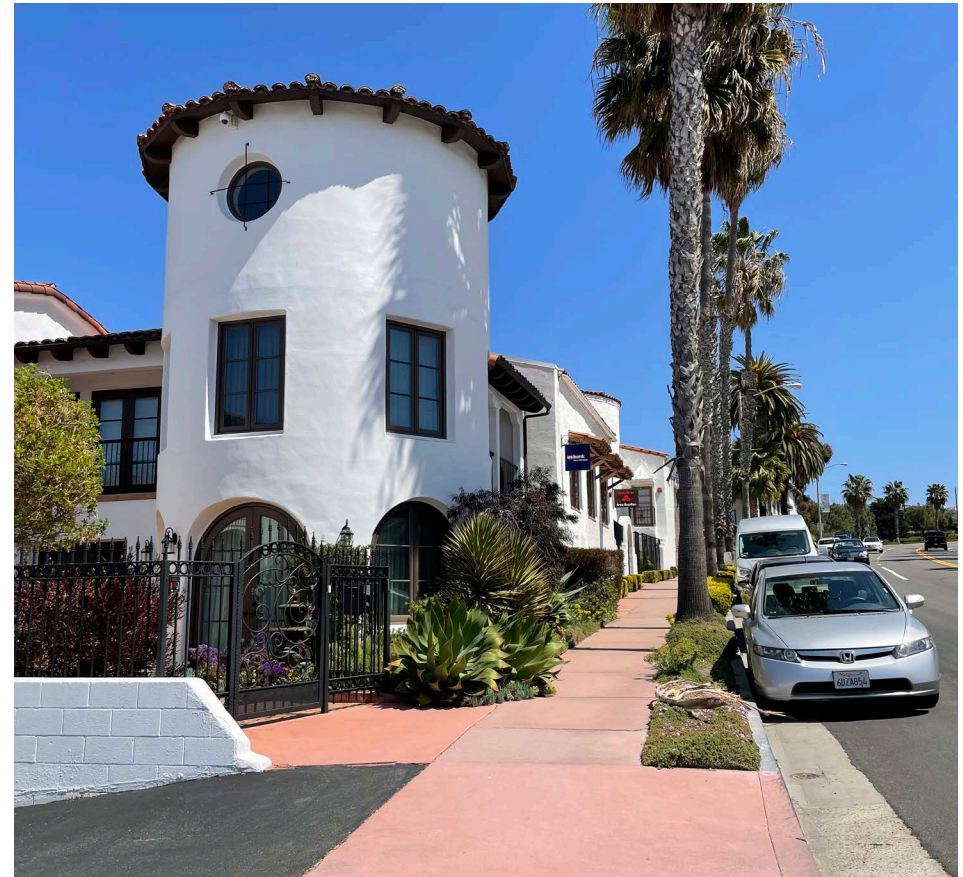
Portion of El Camino Real with landscaped parkway, on-street parking, and engaging building frontages
