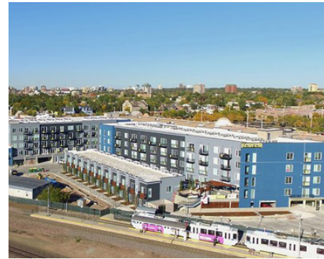
Transit-oriented housing development near light rail
