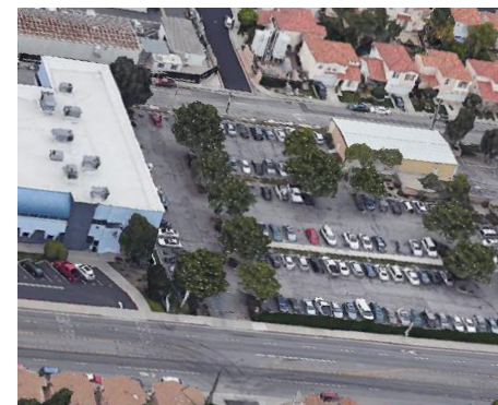
Existing parking lot
