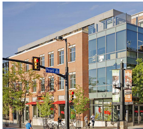
Mixed use retail and office building in Boulder, CO; Source: Nicholas Partnership
