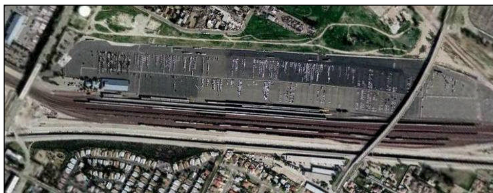
Exhibit 66: BNSF Auto Facility, San Bernardino
