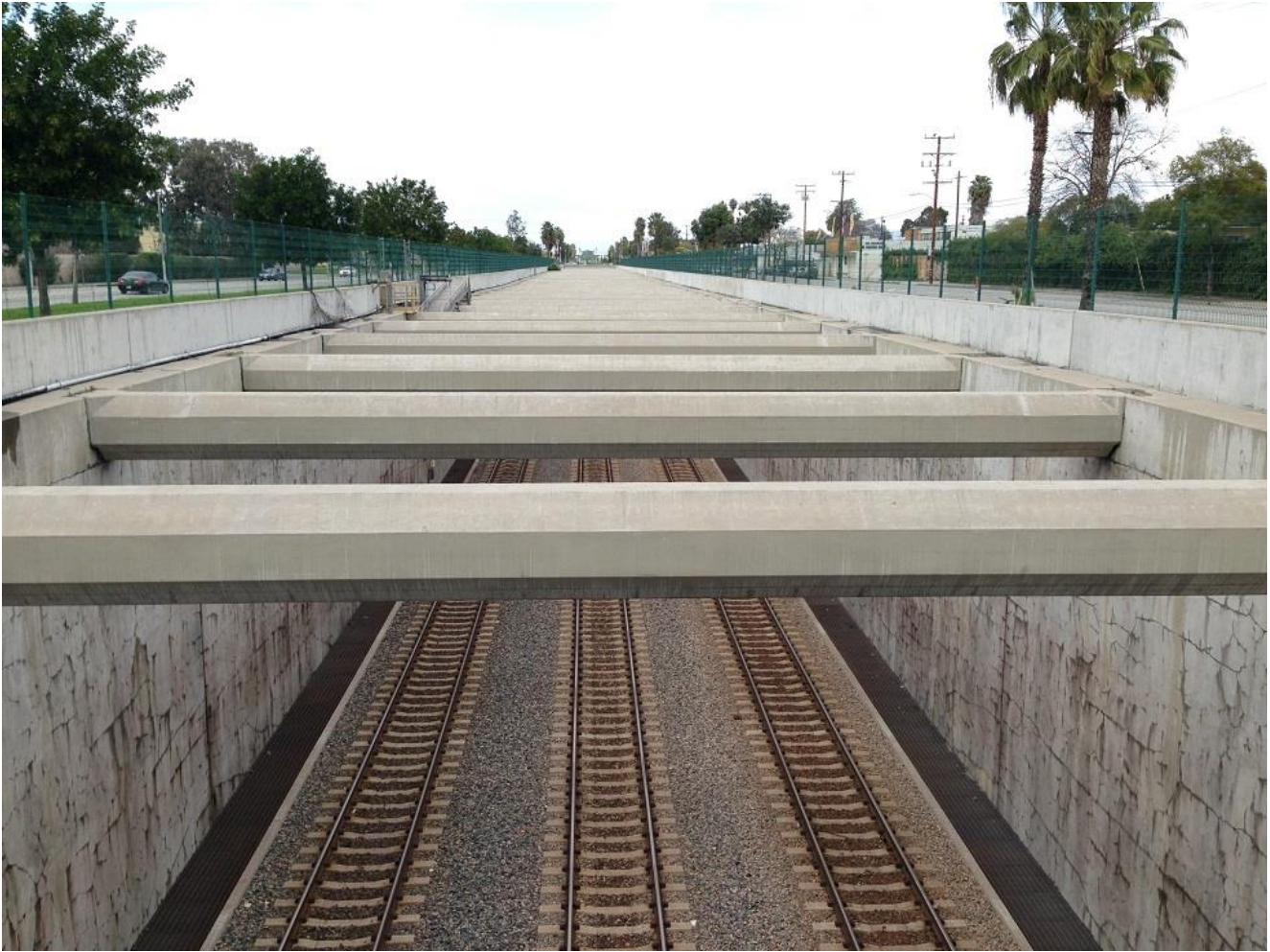
Fig. 6. A section of the Alameda Corridor's mid-corridor trench in the city of Compton. (Photo by Brian Yanity)
