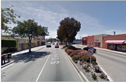
a Existing Condition: Two very wide, fast vehicular lanes northbound and southbound, armored raised medians with Australian Paperbark trees, no on-street parking, and sidewalks in most cases either obstructed and lifted by very large Ficus trees or lacking street trees entirely.
