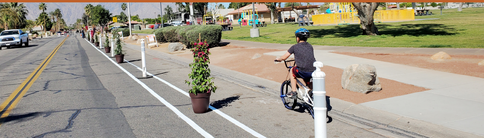
2 A separated bike lane was installed on Tachevah Drive, between Panorama Park to Avenida Maravilla, fronting the park (northside of Tacheva).
