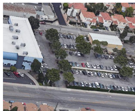
Existing parking lot
