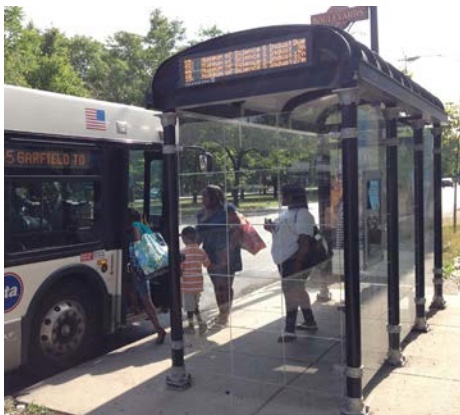
CTA Transit Shelter, Chicago, IL
