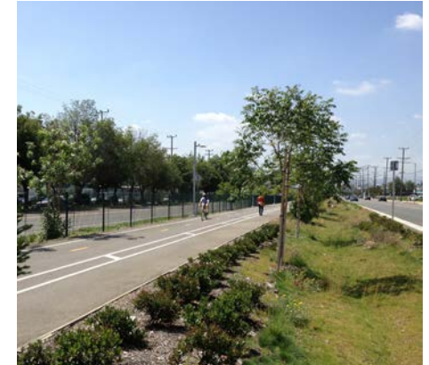
Orange Line Busway, Chatsworth, CA
