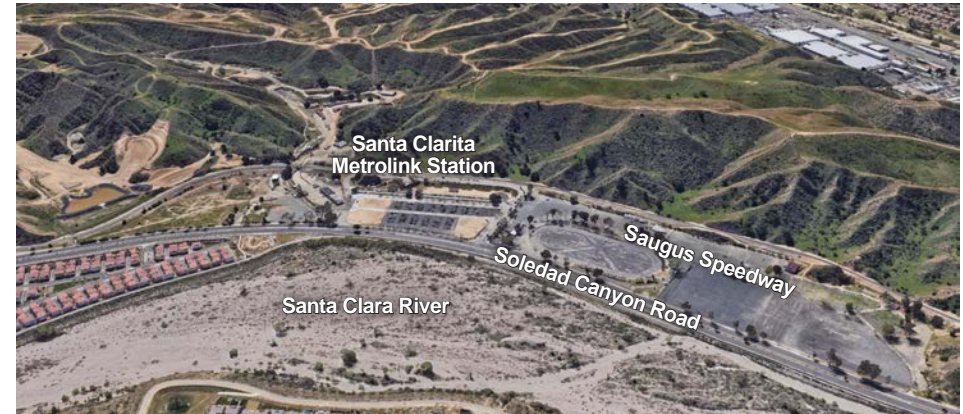
2018 aerial imagery of Subject Area; Source: Google Earth
