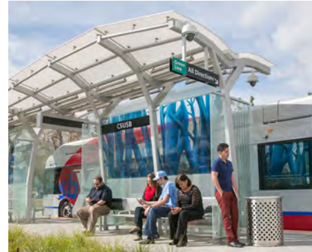
sbX Transit Shelter, San Bernardino, CA
