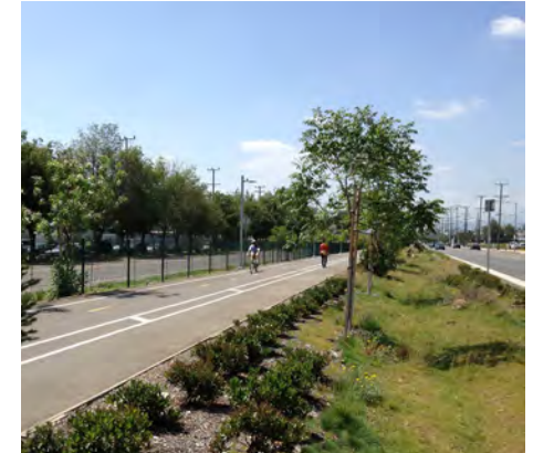
Orange Line Busway, Chatsworth, CA
