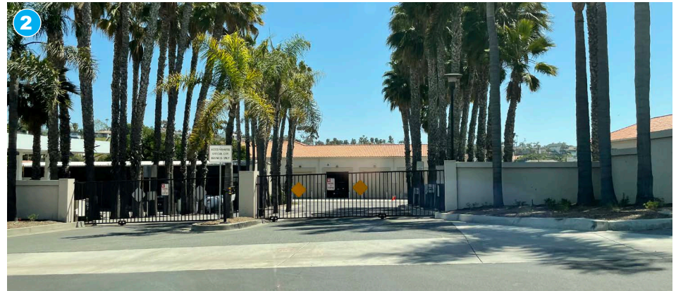
Water reclamation plant
