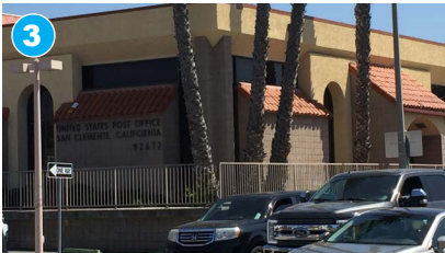
Post office fencing Avenida Pico
