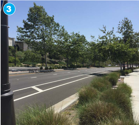
Bicycle lanes and pedestrian improvements on Avenida Vista Hermosa
