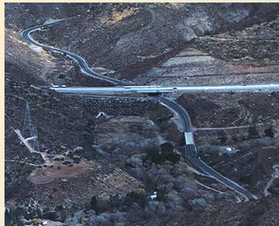
Agua Dulce Canyon vehicle underpass, with drainage culvert for stream visible to the left of the underpass.
