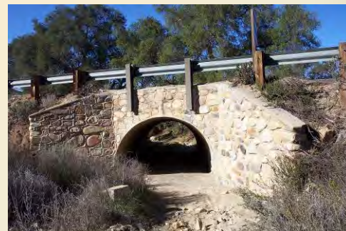
Kolb Creek bridge on the SR-79.
