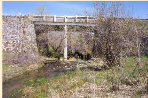
Bridge for Santa Ysabel Creek on SR-79.
