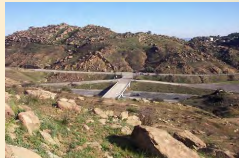
Looking south at the Rocky Peak overpass.
