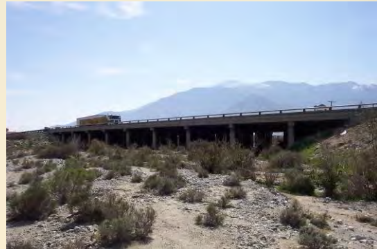
Bridge spanning the San Gorgonio River.
