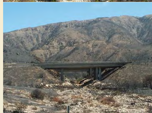
Bridges on I-15 north of Cleghorn Canyon; the top is 0.7 miles north of Cleghorn; the bottom is 400 yards south of the Cajon interchange.
